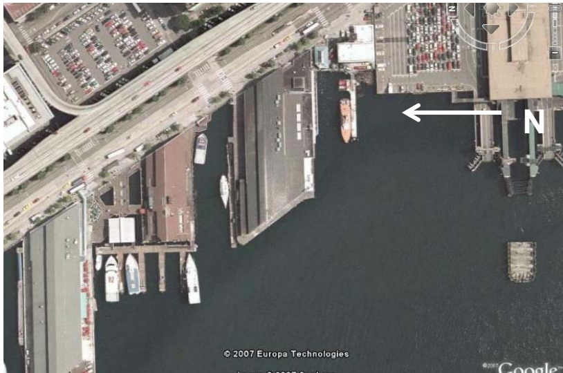
Figure B-4. Aerial view of Pier 55-56.
