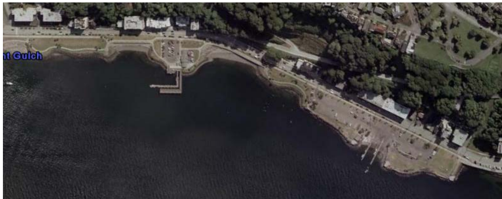
Figure B-3. Aerial view of Seacrest Pier and surrounding area.
