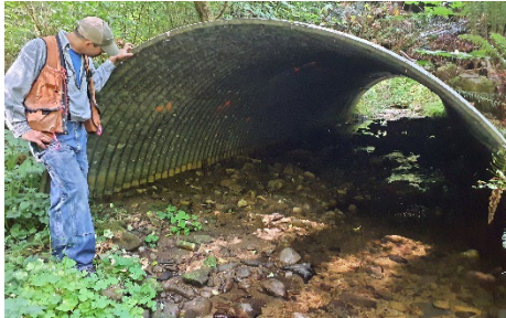
Improving Aquatic Organism Passage. Culvert replacements like this one on Warner Creek (Astoria District) improve aquatic organism passage, which increases habitat accessibility and habitat
