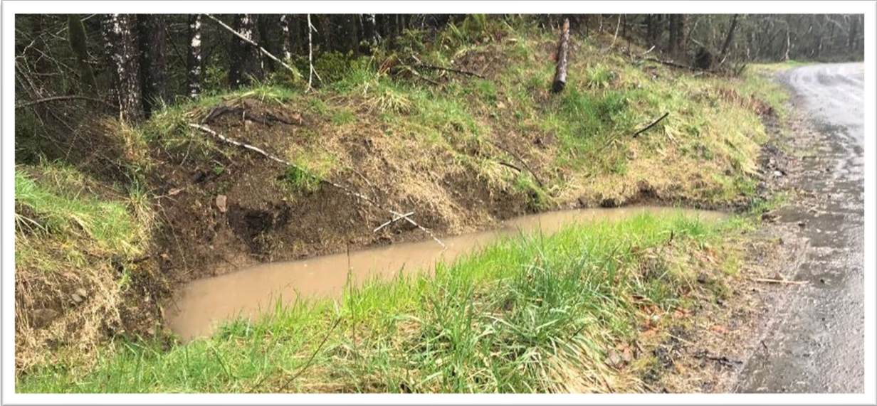
Photo 1. Example of other measure, settling basin.
