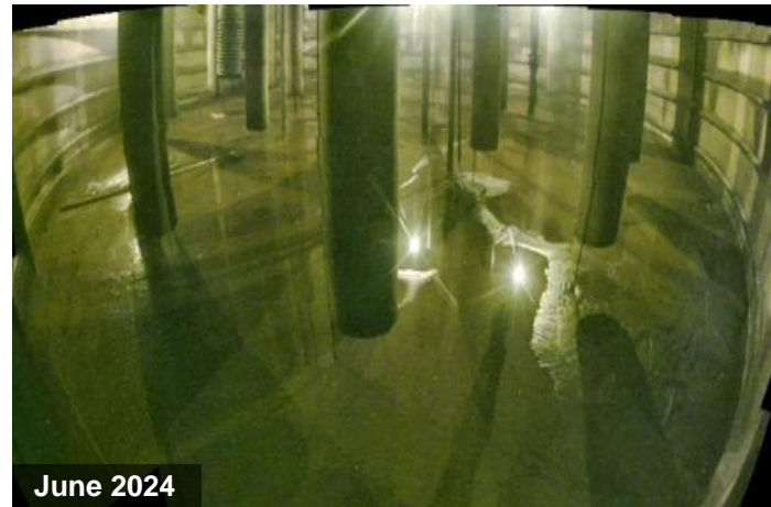
Tank AX-101 after retrieval of approximately 346,000 gallons of waste
