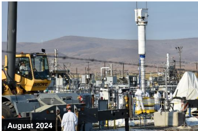
Test Bed Initiative mast being lowered into Tank SY-101
