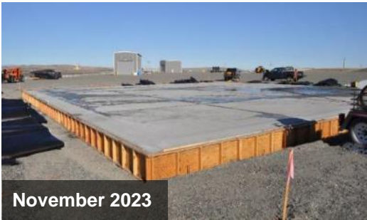
Recently constructed 80-by-80-foot concrete pad at the Integrated Disposal Facility
