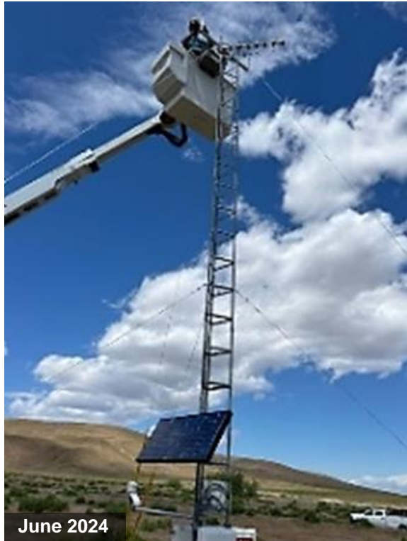
Crews inspect and repair Hanford Site meteorological towers
