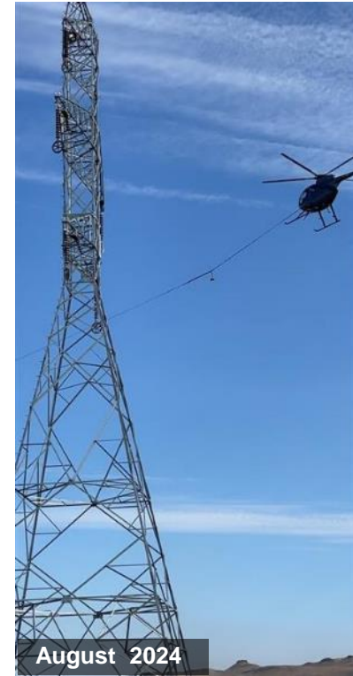
Helicopter pulling electrical cable
