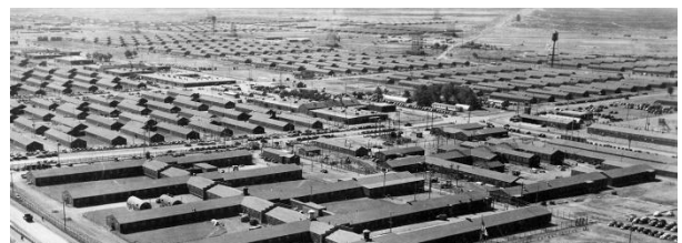
More than 50,000 construction and tradespeople lived in make-shift camps on the site. Very few of them knew the totality of the project they were building.
