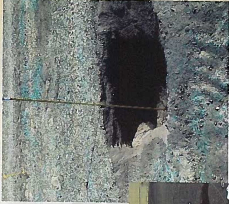
216-C-9 crib collapse
