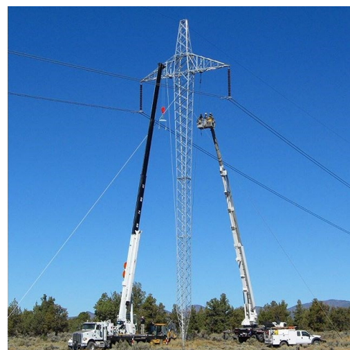
Crews from Central Electric Cooperative perform maintenance and repairs on high-voltage lines.
