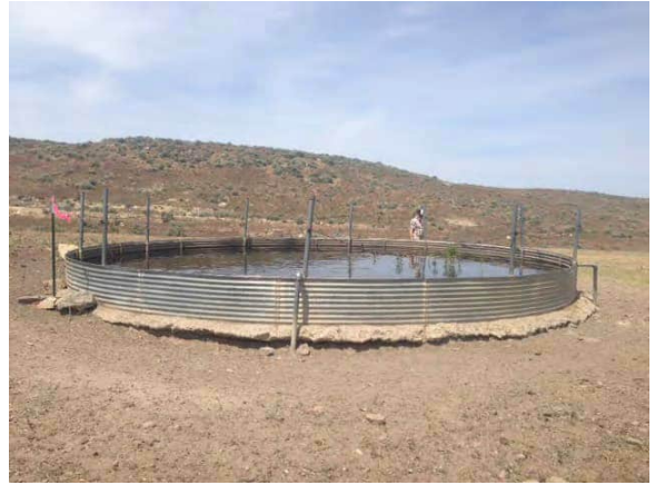
Photo A-18. Grassy Springs Stock Tank
