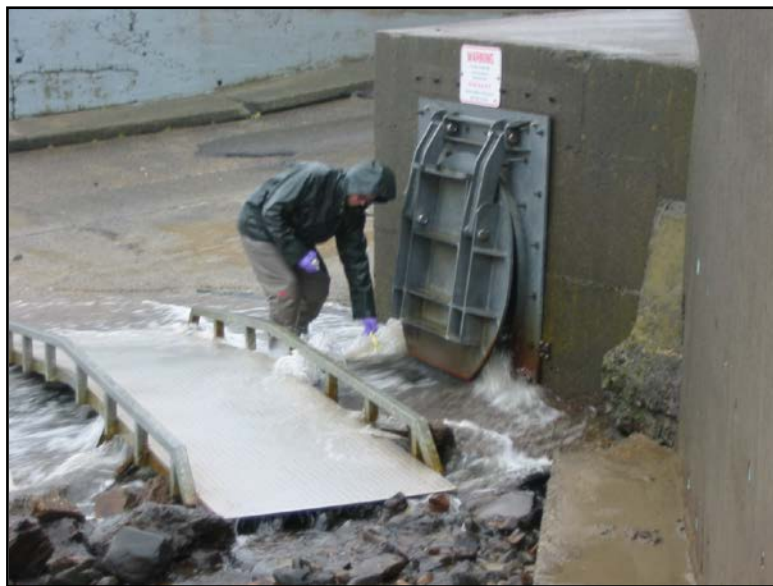
Figure 23. Gower Street Creek at the Ecola Court outfall.
