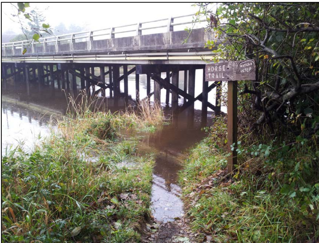
Figure 16. Ecola Creek at the Fir Street Bridge.
