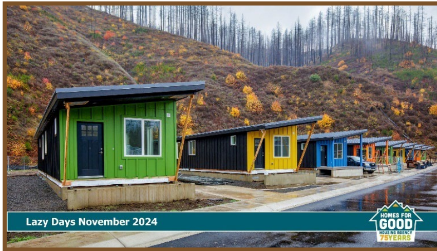
Photo of newly installed homes at the Lazy Days MHP
