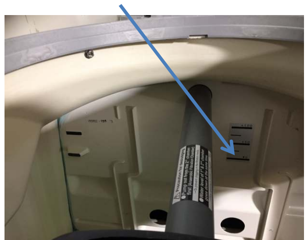
Low water line in sedimentation chamber
