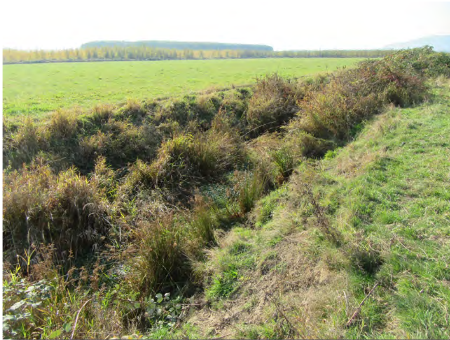
PHOTOGRAPH 18 - Looking west along the ditch at the southern edge of the study area. Photograph taken by Sue Brady on October 22, 2018.
