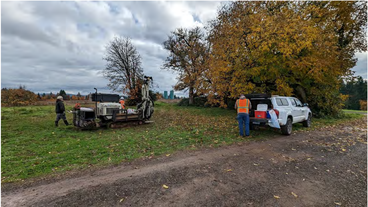
Photo 3. Looking southeast toward a direct-push drill rig.
