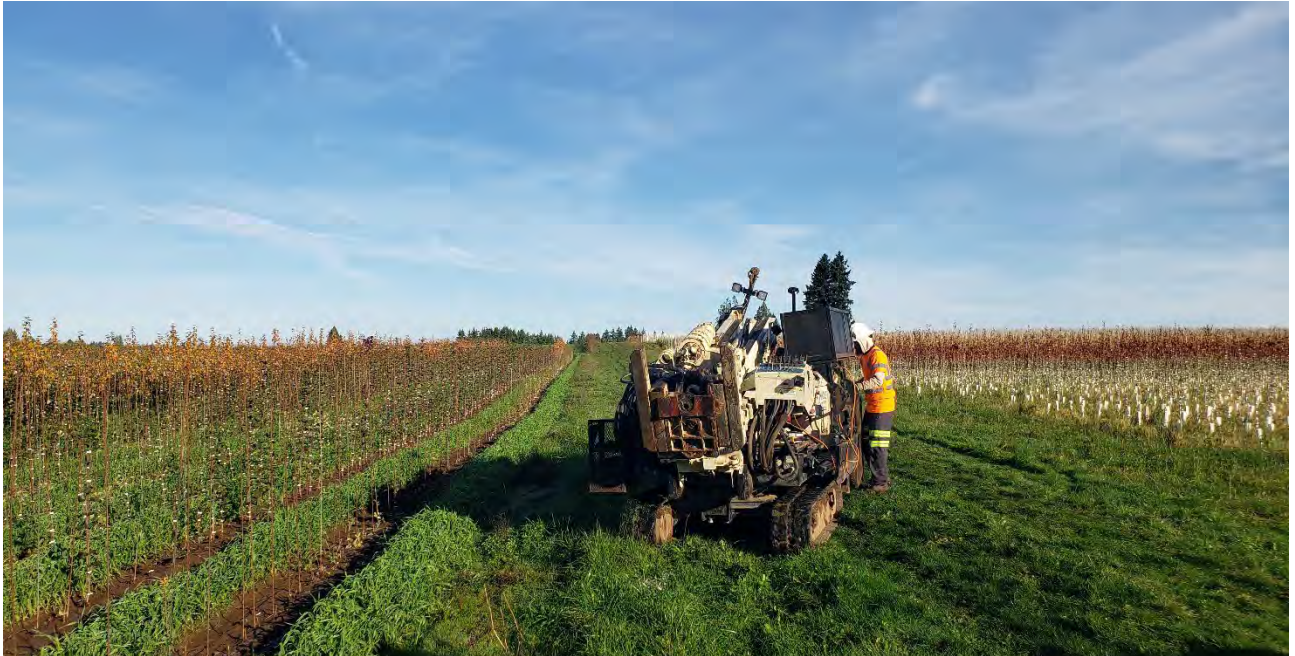
Photo 5. Looking north at the Finished Water Center assessment location.
