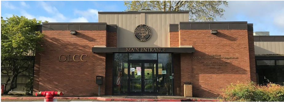
OLCC Headquarters – McLoughlin Blvd.
