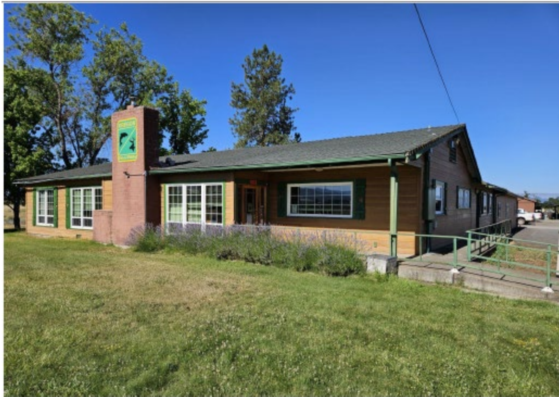
Exterior of the main office at Denman Wildlife Area.
