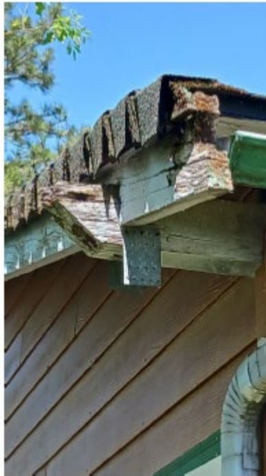
Pictures showing typical rot conditions of the building exterior, water staining on the ceiling from leaks, and a rotting single pane window.
