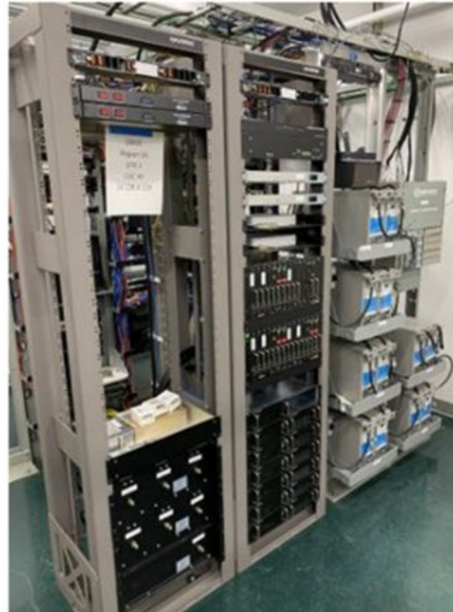
CDC radio tower & P25 radio system
