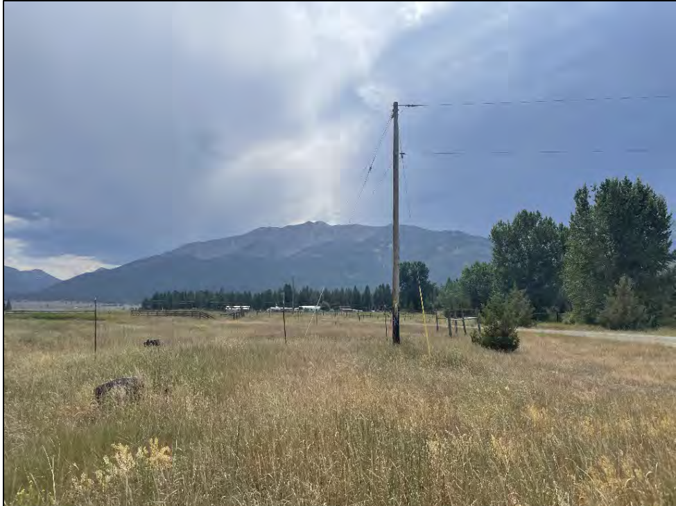
Photo 3. Looking south at the obstruction power pole and dense grasses.
