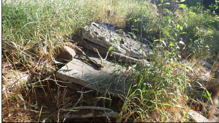
Figure 4-8. Concrete along the west bank of Hurricane Creek representing the remnants of the former milking parlor.
