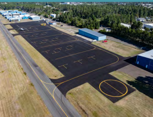
Florence Airport Pavement Rehab
