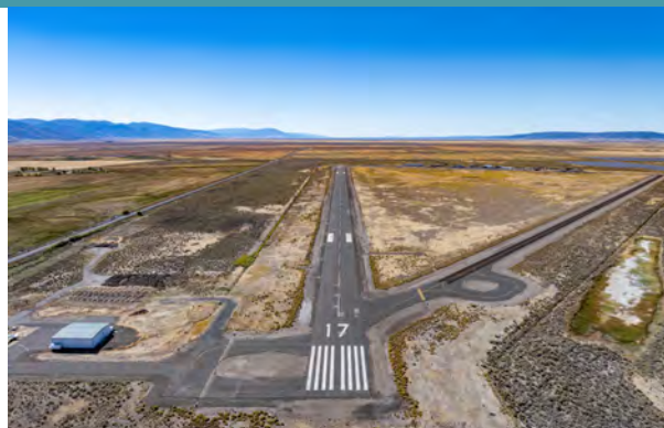
Lakeview Taxiway Rehab
