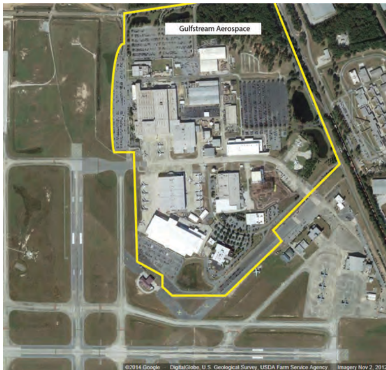
FIGURE 1-9: Savannah/Hilton Head International Airport
