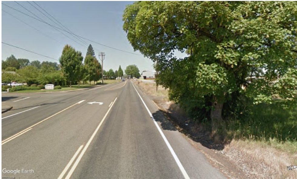
Figure 1: DFI No. D01535, looking West
