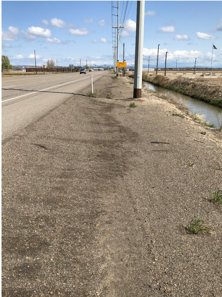
Figure 1: DFI No. D01488 looking North
