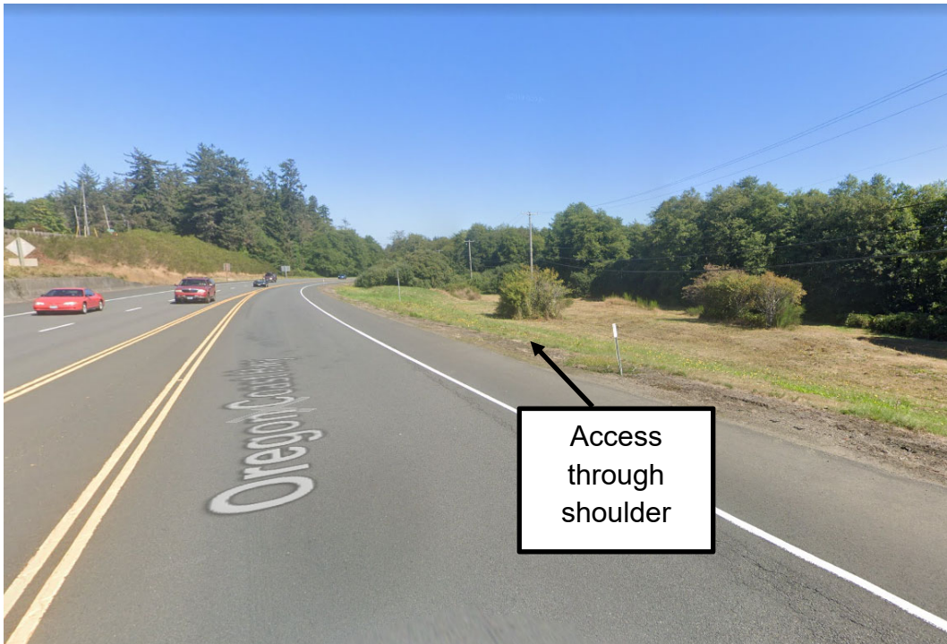
Figure 3: Access along the shoulder
