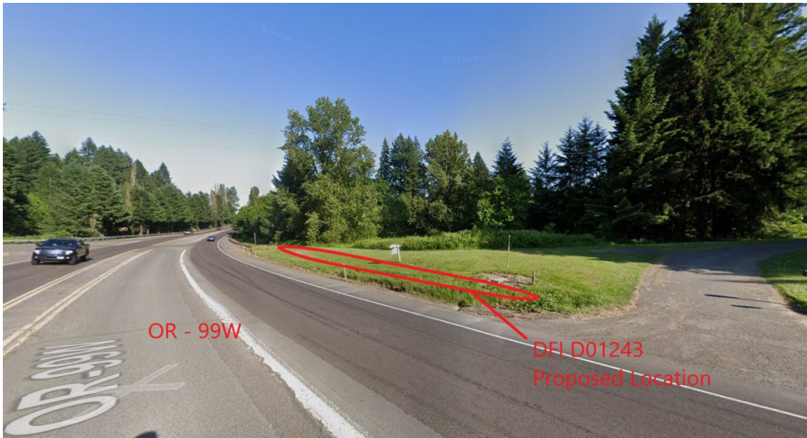
Figure 1: DFI No. D01243, looking east (existing condition)
