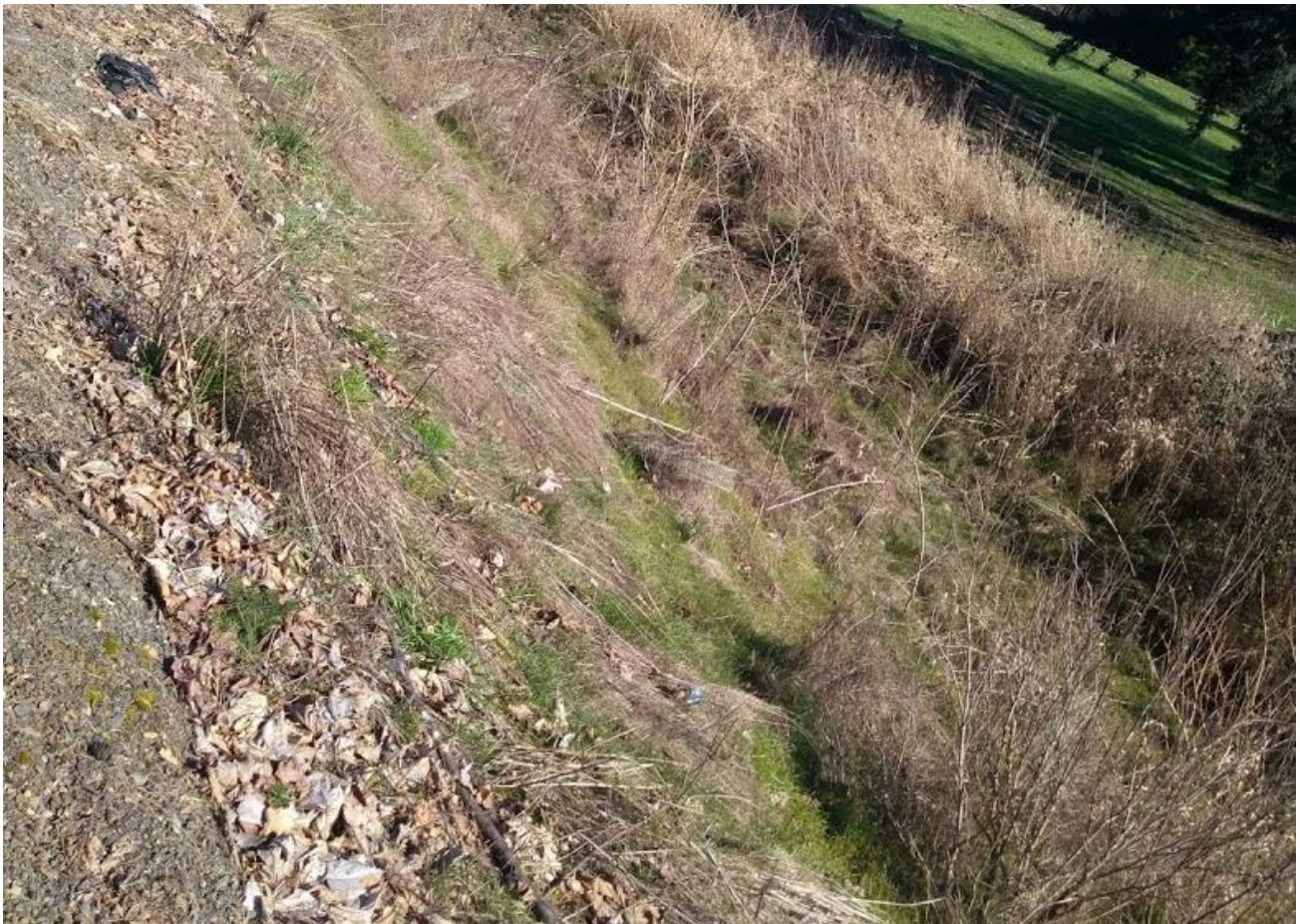
Figure 1: DFI No. D01228, looking southeast
