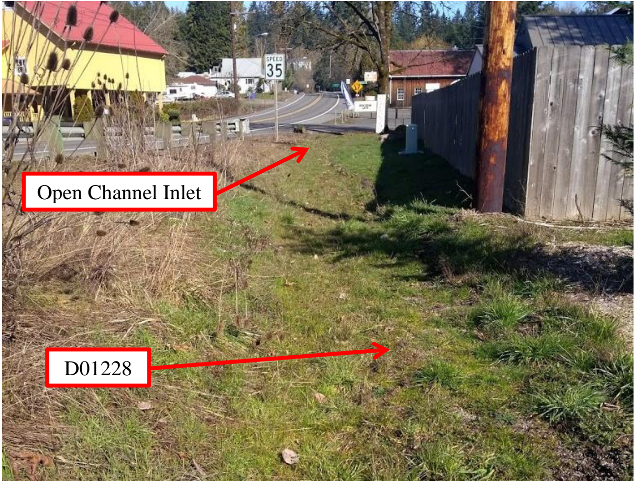
Figure 4: Beginning of the water quality facility, looking north
