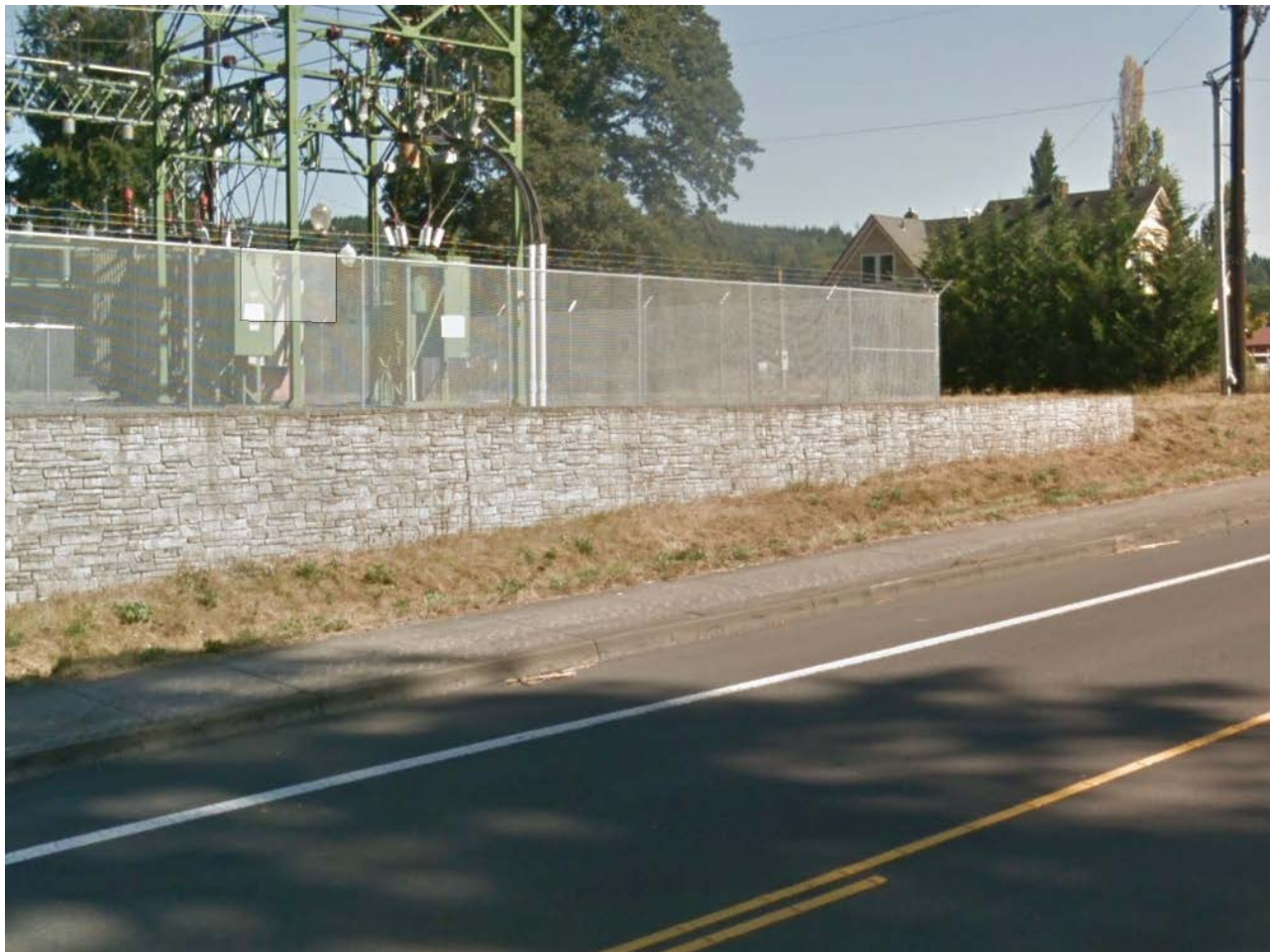
Figure 1: DFI No. D01226, looking southeast
