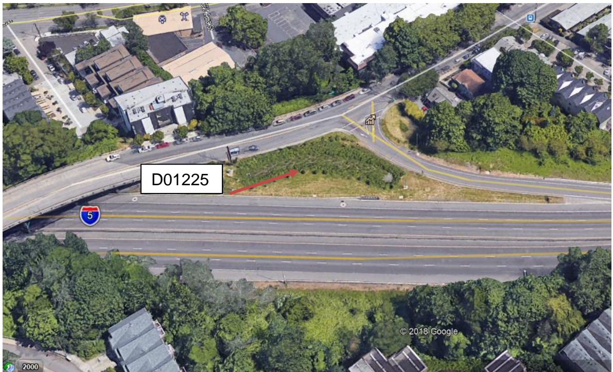
Figure 1: DFI No. D01225, looking southeast
