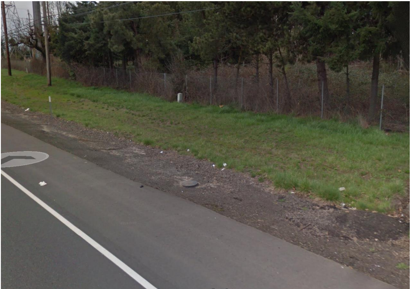
Figure 1: DFI No. D01219, looking south
