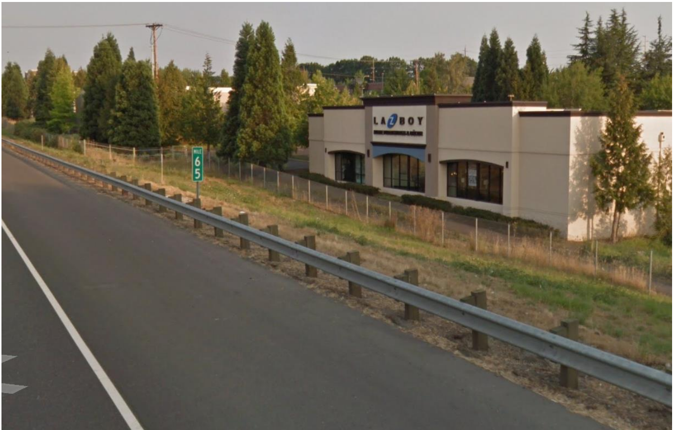
Figure 1: DFI No. D01218, looking southeast
