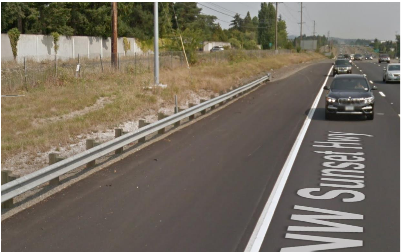
Figure 1: DFI No. D01215, looking east
