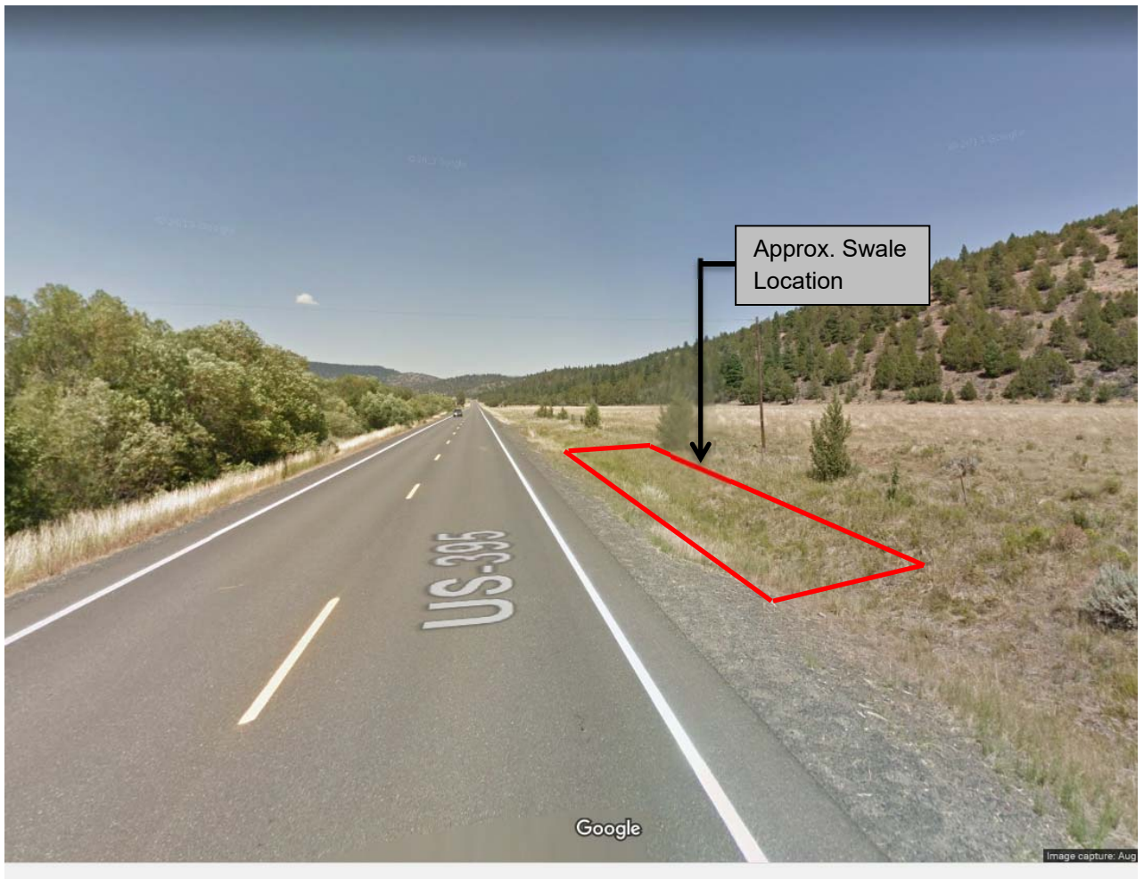
Figure 1: DFI No. D01213, looking North
