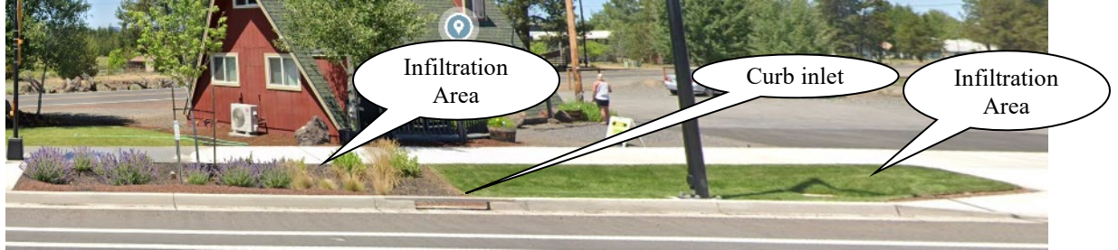
Photo 1: Infiltration area at MP 168.05.
