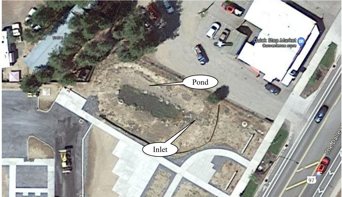
Photo 1: Infiltration area designed to infiltrate the 100 year storm, thus there is no outlet.
