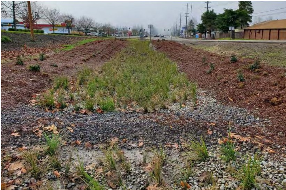
Figure 1: DFI No. D01120, looking South
