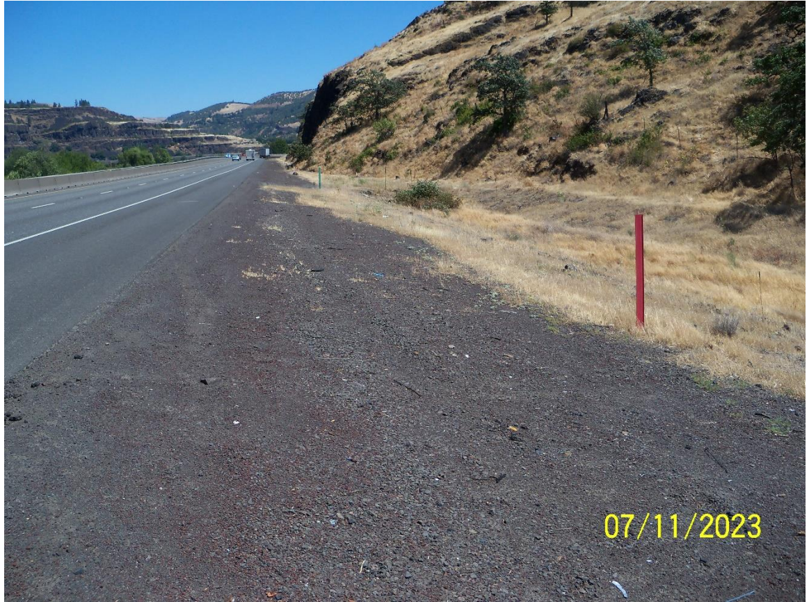
Figure 2: Access from shoulder of 84-East
