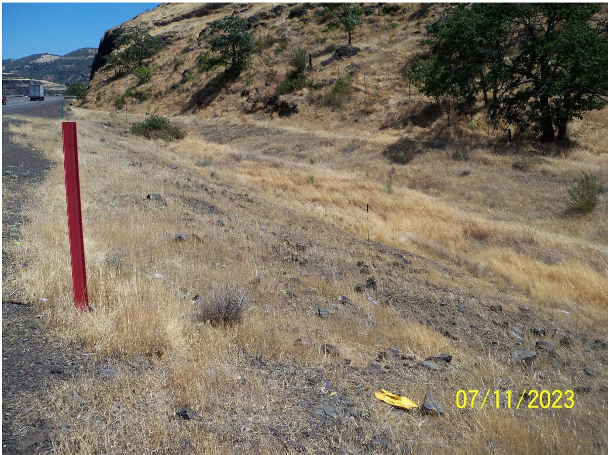
Figure 1: DFI No. D01117, looking east at facility from 84-East shoulder
