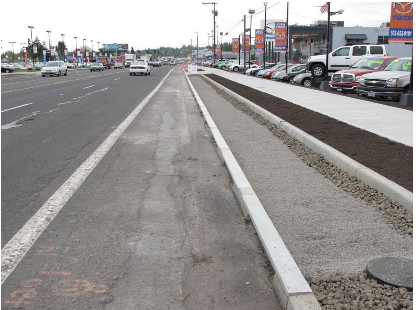
Figure 1: DFI No. D01056, looking south
