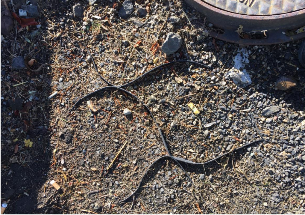
Figure 7: Cellular Confinement Grid with ecology mix
