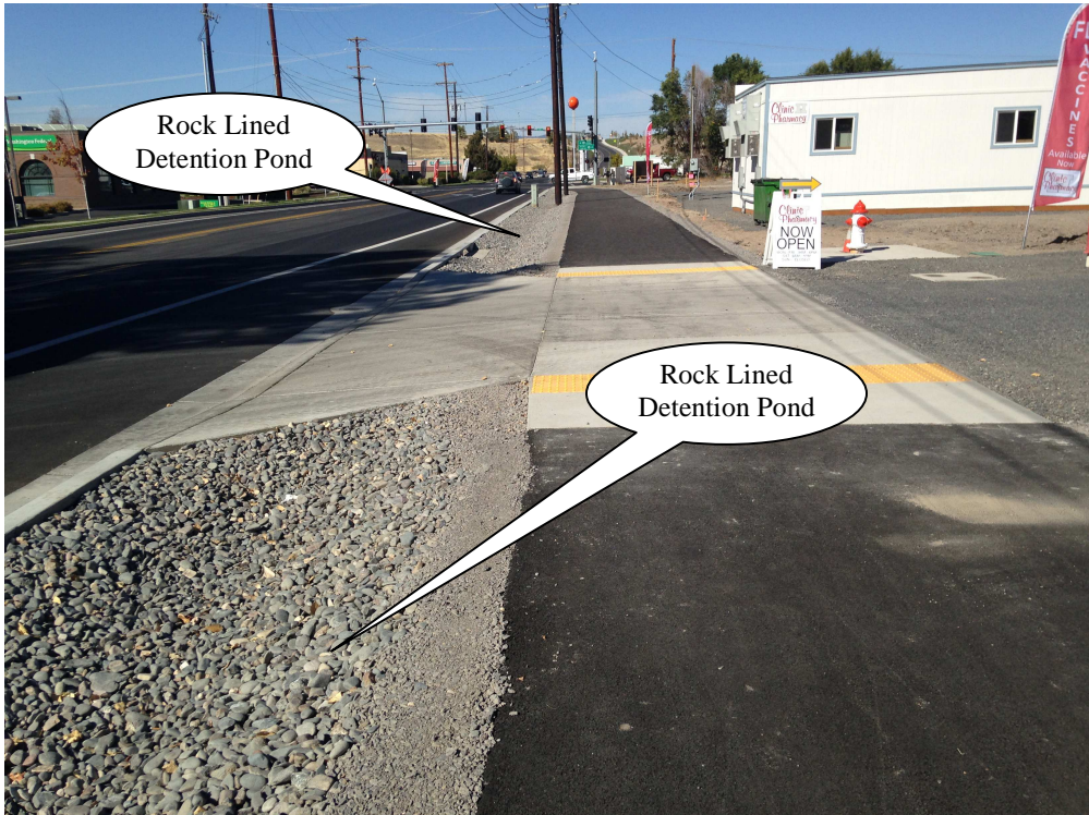
Photo 1: Detention pond facility looking north toward 3 rd Street (US HWY 26).
