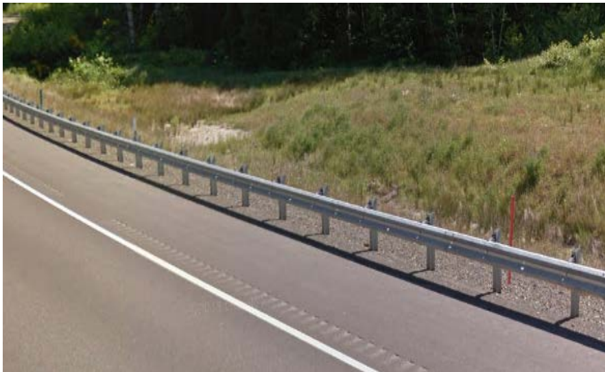
Figure 1: DFI No. D00972, looking south
