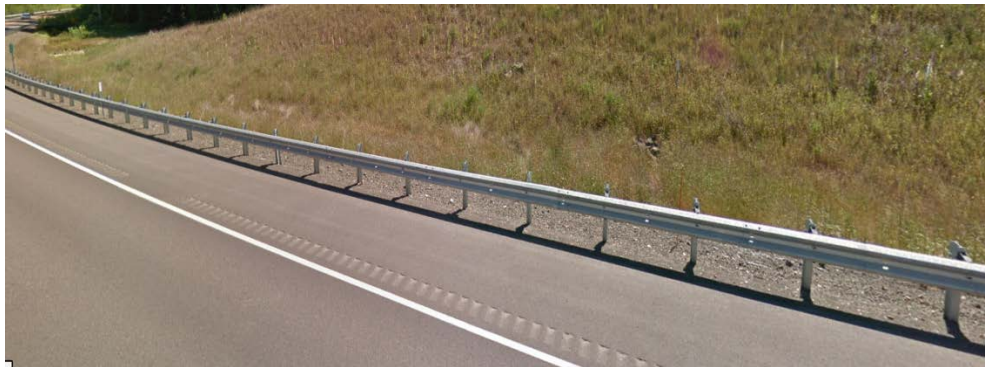
Figure 1: DFI No. D00971, looking east
