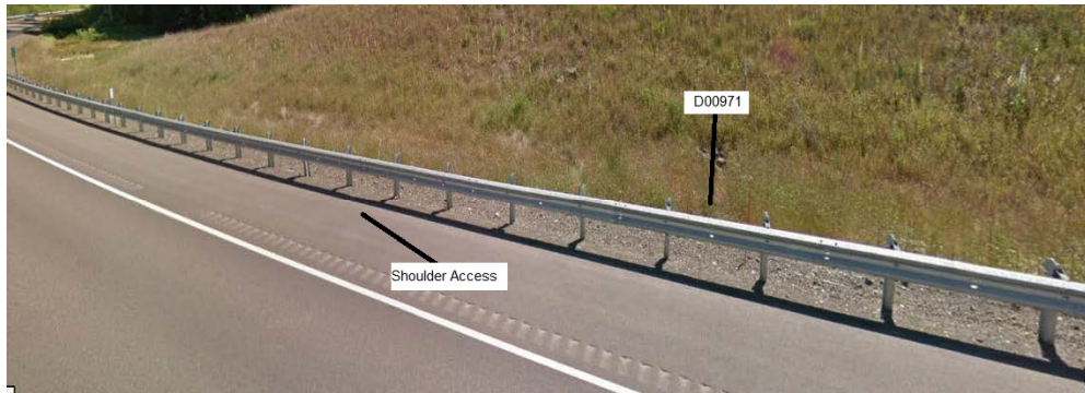
Figure 3: Highway No.: 33, looking east
