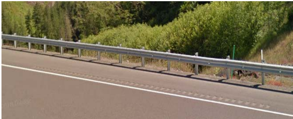
Figure 1: DFI No. D00968, looking east
