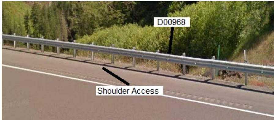
Figure 3: Highway No.: 33, looking east
