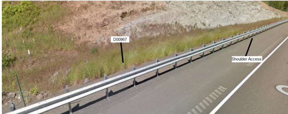
Figure 3: Highway No.: 33, looking east
