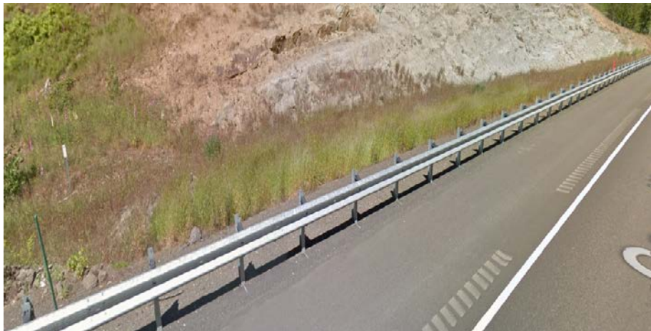
Figure 1: DFI No. D00967, looking east
