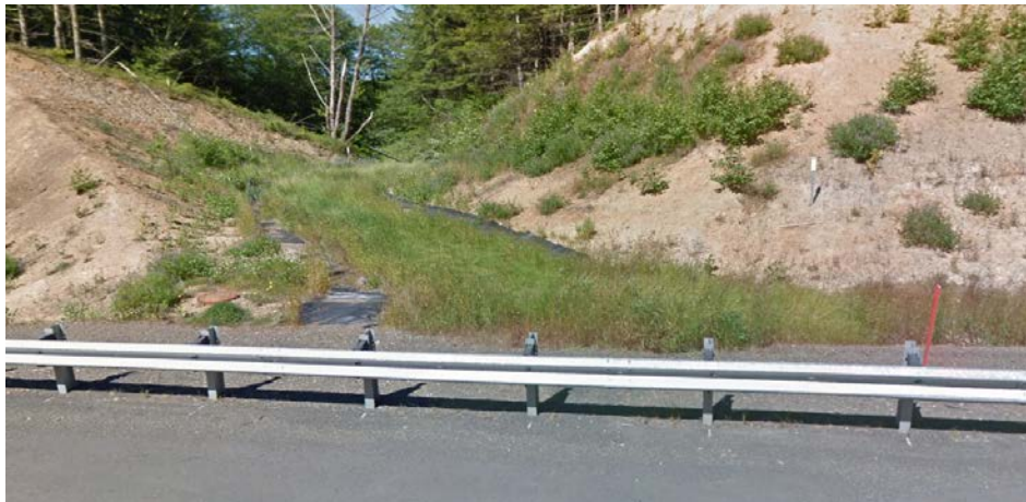
Figure 1: DFI No. D00965, looking north
