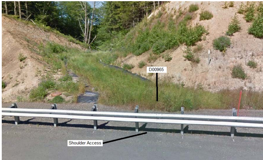
Figure 3: Highway No.: 33, looking north
