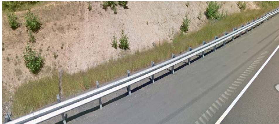
Figure 1: DFI No. D00964, looking east
