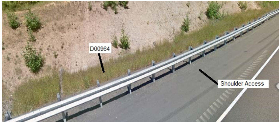
Figure 3: Highway No.: 33, looking east
