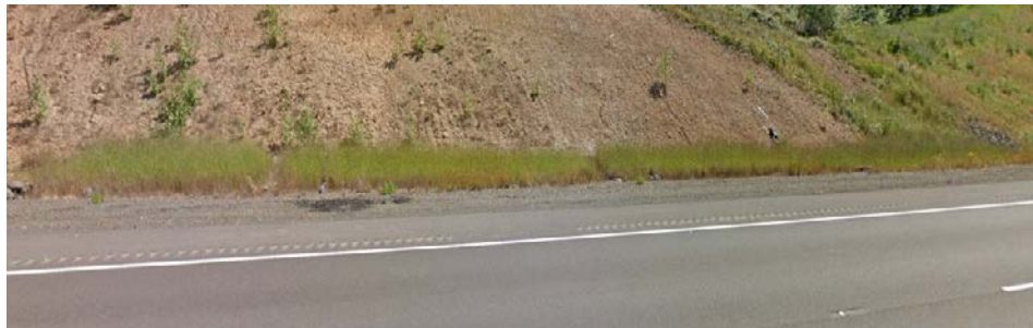
Figure 1: DFI No. D00963, looking west
