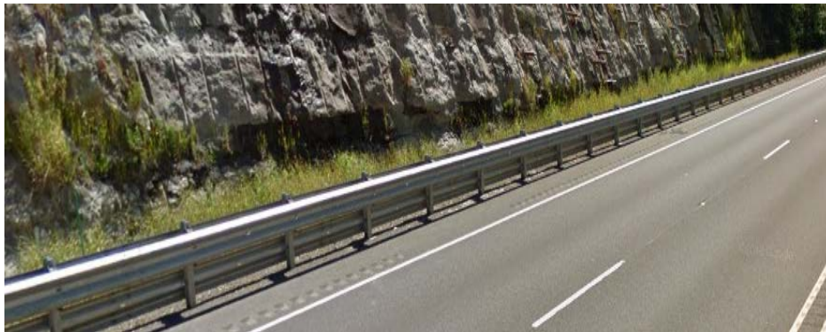
Figure 1: DFI No. D00962, looking west
