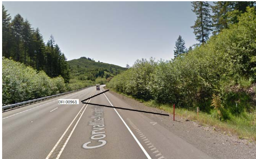
Figure 1: DFI No. D00961, looking [west]
