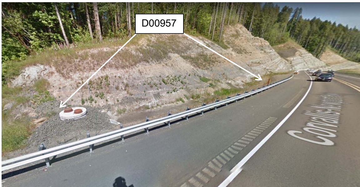
Figure 1: DFI No. D00957, looking East
