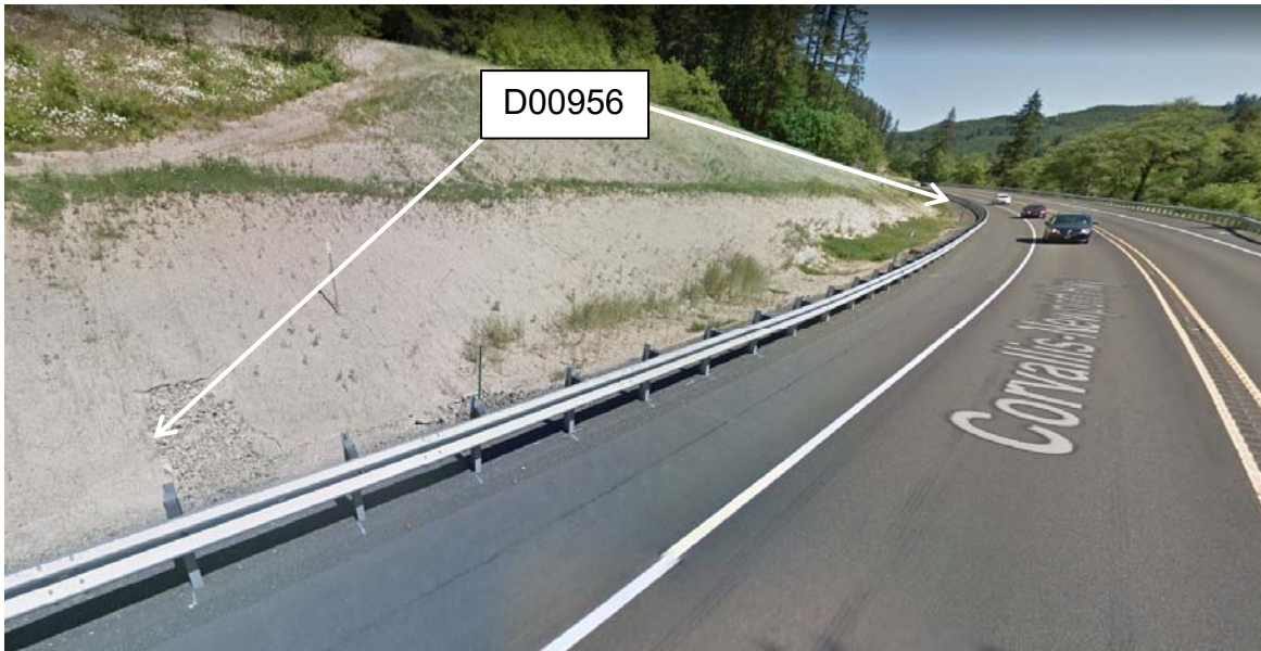
Figure 1: DFI No. D00956, looking Southeast
