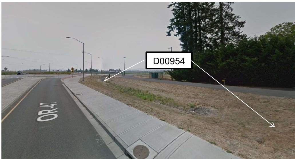
Figure 1: DFI No. D00954, looking South
