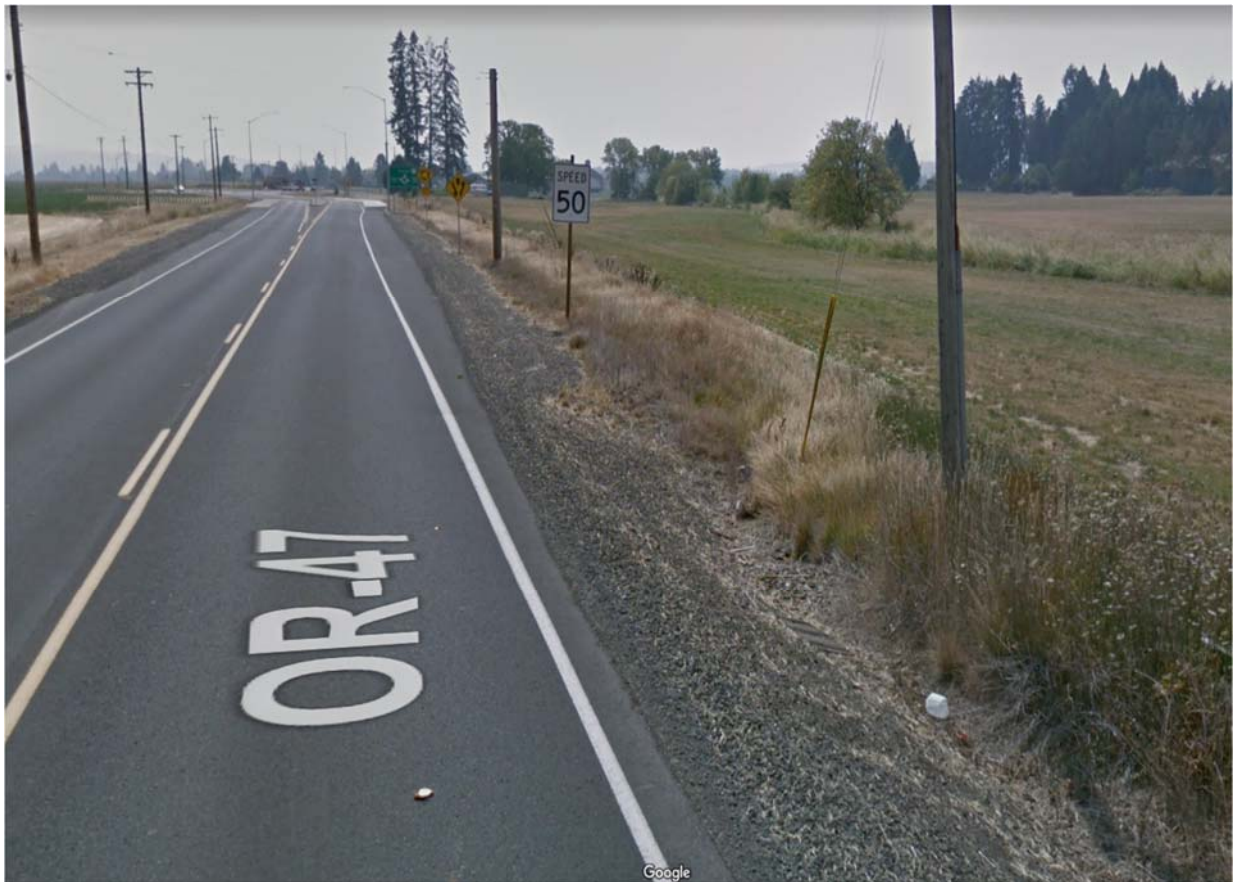
Figure 4: DFI No. D00952, looking South on OR47, roadside shoulder access
