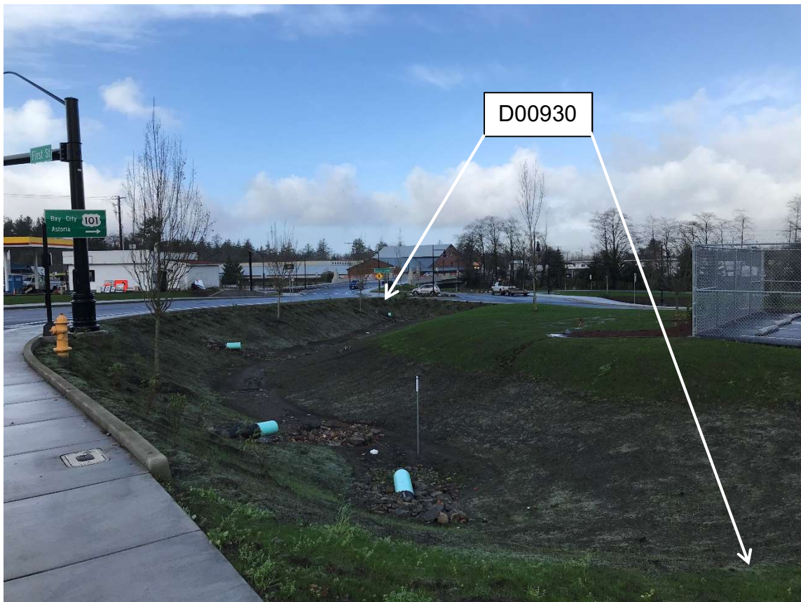
Figure 1: DFI No. D00930, looking North
