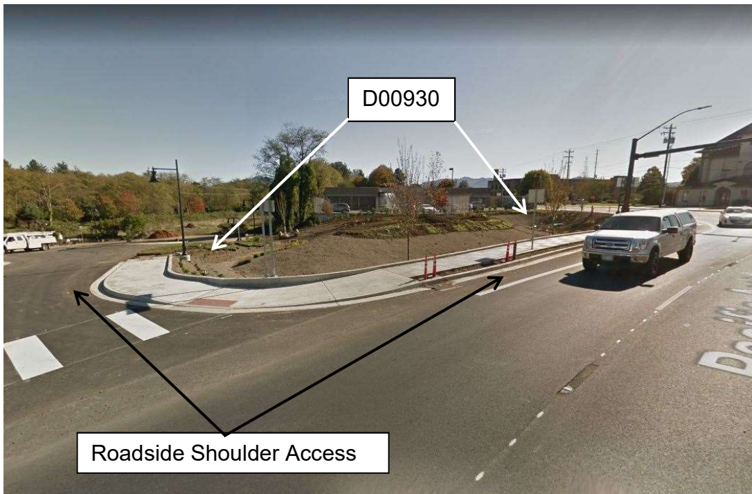
Figure 3: D00930, Looking Southeast
